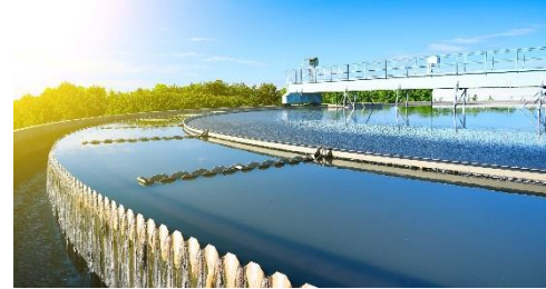
WATER UTILITIES & SERVICES
